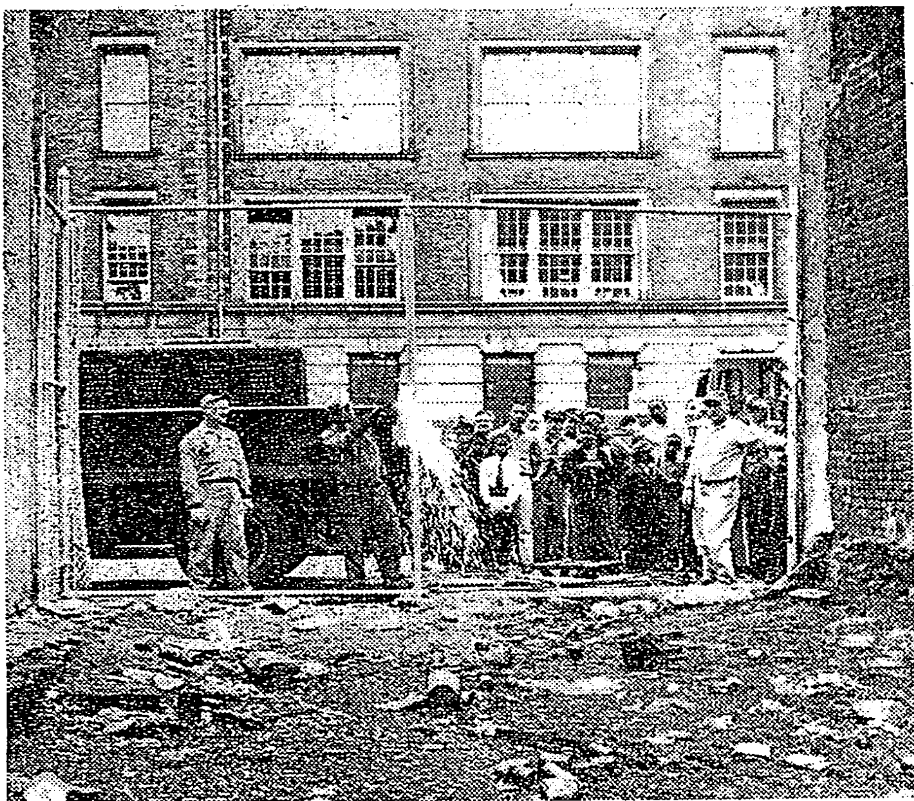
Welder cuts part of fence on St. Nicholas Avenue to permit a Department of Sanitation cleaning force to pick up the trash and move in topsoil.
